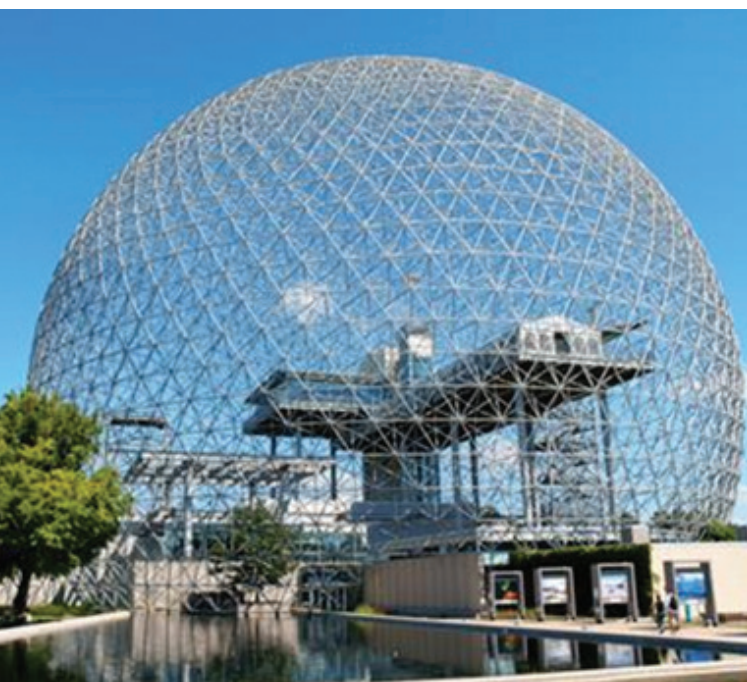
Figure 1 Buckminster Fuller geodesic dome, the USA pavilion in Montreal exhibition 1967, is a structure which was inspiration, as mimicry, to Kroto who named molecule C_{60} : fullerene. Icosahedron is composed of 20 triangles and Buckminster cupola is composed of 20 \times n triangles as optimization of design, mass and energy (light).
